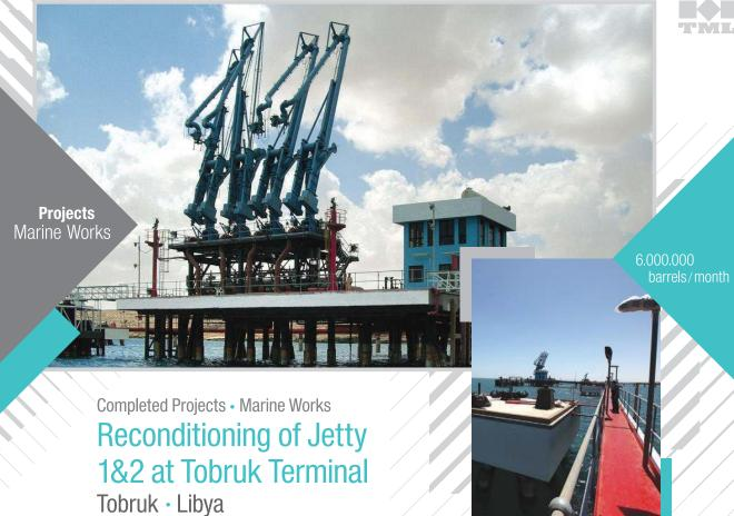
Currently serving as Terminal for Tobruk Refinery of Arabian Gulf Oil Company (AGOCO), the Jetty's construction had started in 1964 and was officially inaugurated by exporting the first shipment of crude oil from Sarir fields in 1967 by accommodating 65.000 DWT tankers. Its design was upgraded and in 1978, it was re-constructed to accommodate tanks up to 150.000 DWT.
